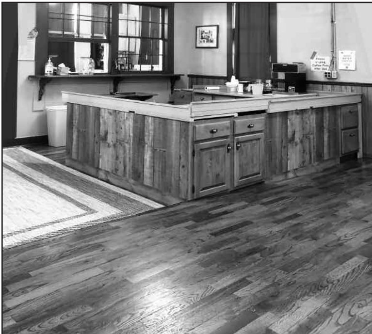
New serving center cabinets installed, awaiting countertop completion.
