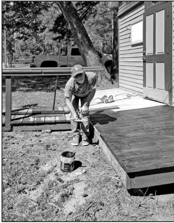
Ken Spoor replaced the front porch at Pleasant Park.
